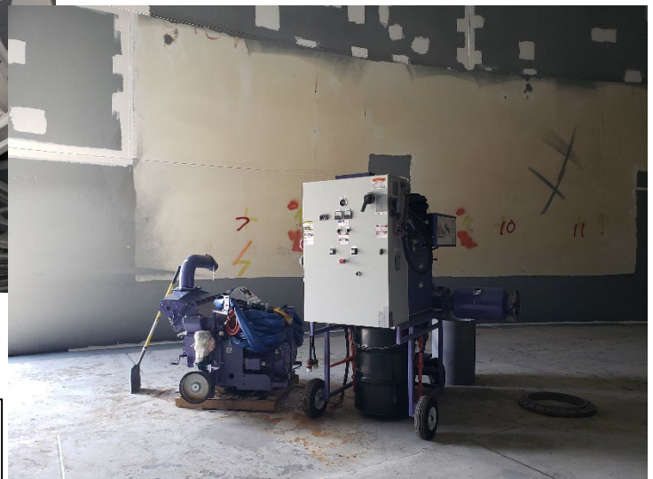
Mobilizing the robotic sandblaster for wall preparation has begun.
