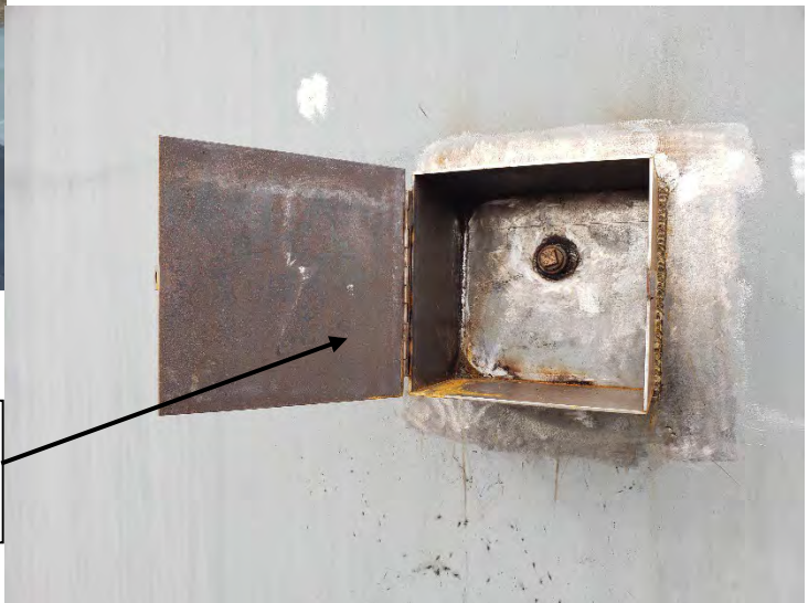
New side mounted lockable sample station. This new feature will substantially reduce operator time for water quality sampling.
