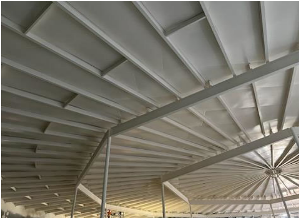
View of ceiling final epoxy coating.
