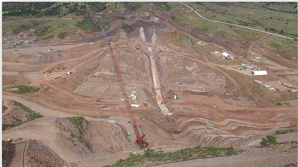
Construction as of July 5
