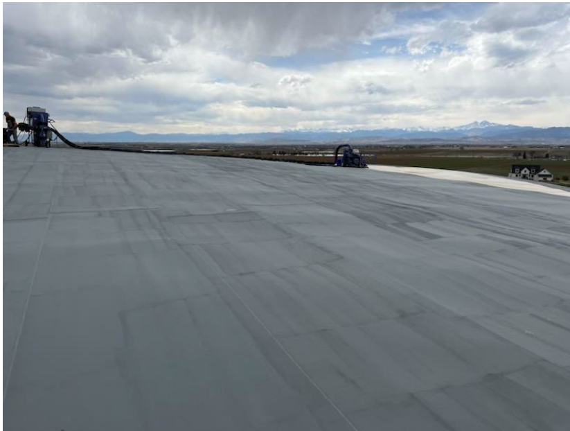
Sandblasting & priming of the exterior nearing completion.
