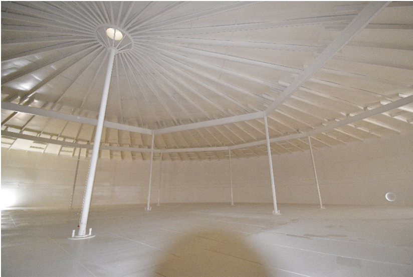
Completed interior coating.
